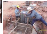
Holding Down Bolt Installation.
