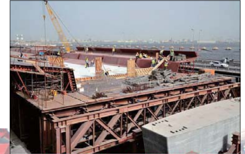
Installation of Formworks at South Marine Bridge (East) (1)
