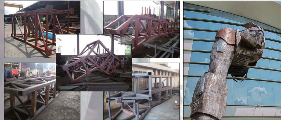
Fabrication in progress.
