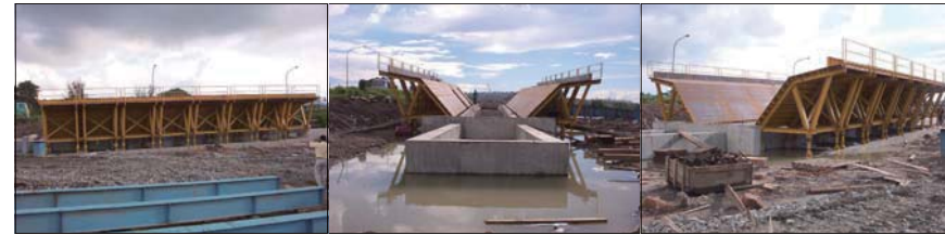
Steel Form Work.
