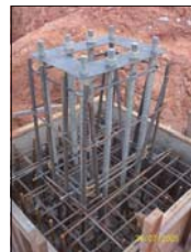
Holding Down Bolt Installation.
