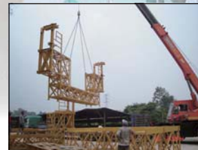
Loading At Our Storage Yard.
