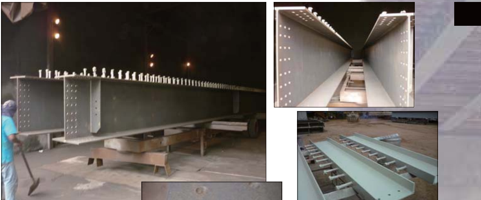
Sand blast & painting In progress.
