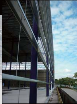
Site erection works.
