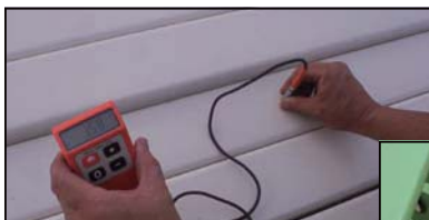
Coating Thickness Check.
