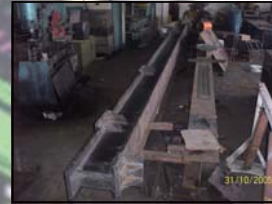
In house Fitting & welding works in progress.
