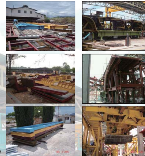
Site Trial Assembly Wing form & Inner core form.
