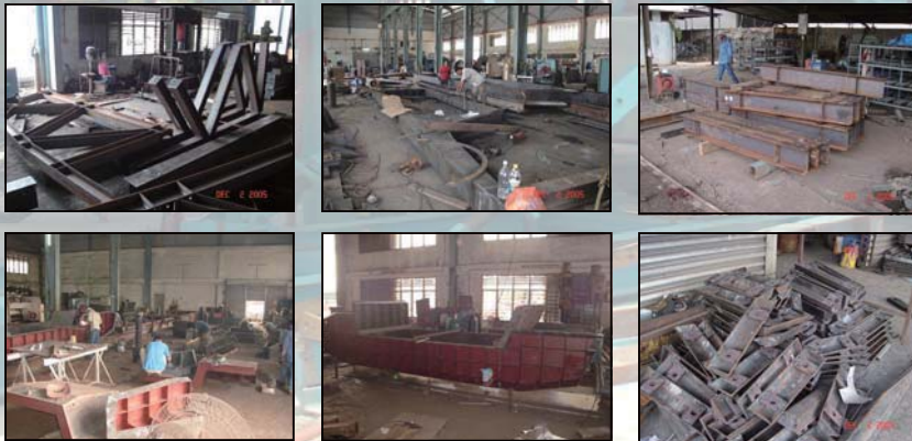
In-house fabrication Wing Form Support and Inner Core Form
