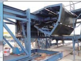
Inner form & hydraulic operation on Site set up.
