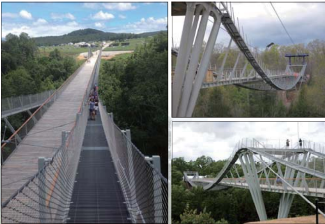
Site erection complete photos.
