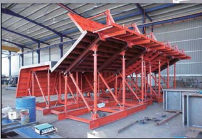
Trial Assembly at workshop.
