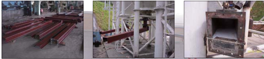
Air Slide - In house fabrication and site installation
