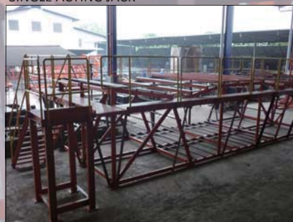
REBAR JIG TRIAL ASSEMBLY
