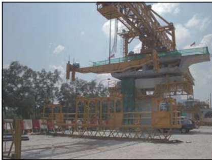
Stressing Gondola , At Site
