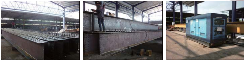
Stud welding on I Girder Beam.
