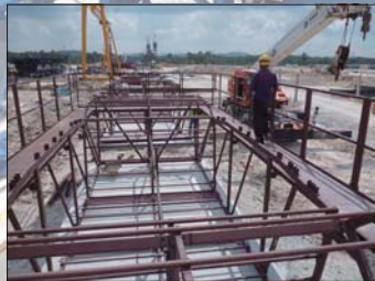
Rebar Jig on Site set up.
