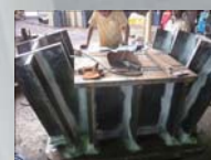
Fabrication In Progress.
