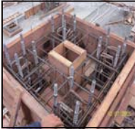
Holding Down Bolts Installation.
