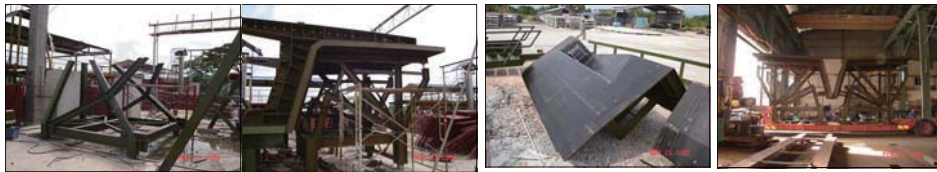
Fit up Inner Core Arm and Wing Form.
