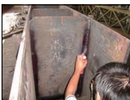
Dye Penetration Test in Progress On Fillet Weld.
