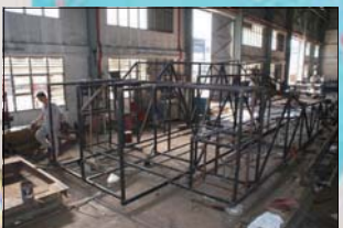
Steel Structure fabrication in progress.
