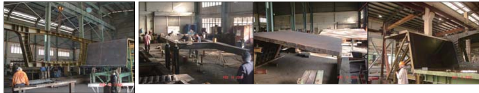
Bulkhead in-house fabrication and trial assembly with wing form.
