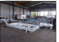
Trial assembly in progress.
