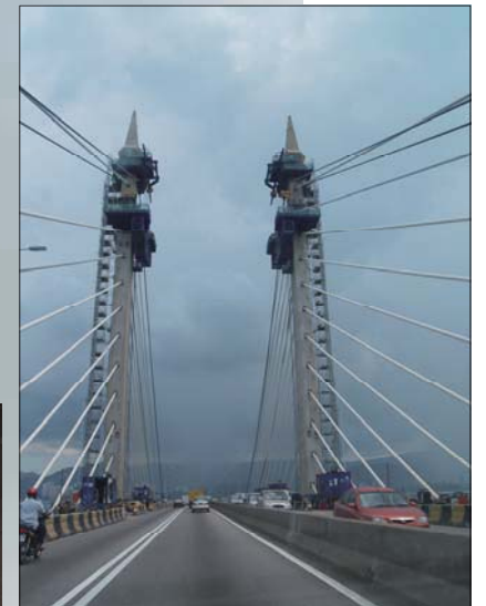
Working Platform Install on Bridge Pylon.
