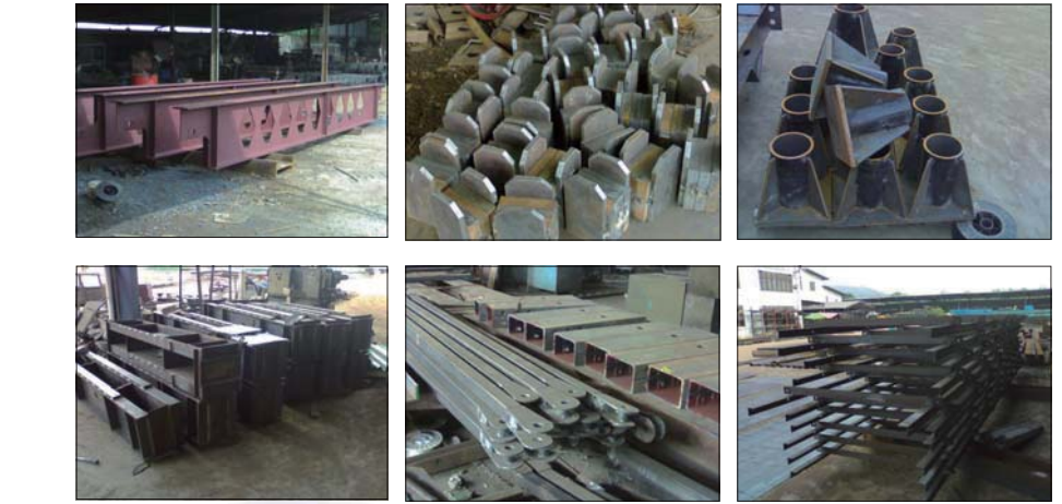
Fabrication in progress.
