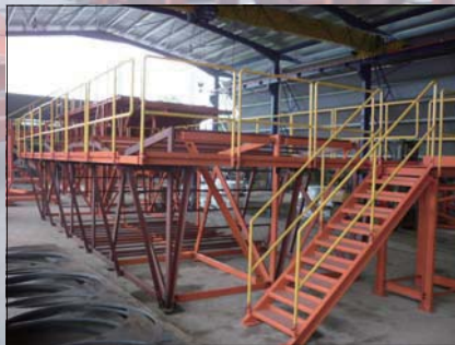
REBAR JIG TRIAL ASSEMBLY
