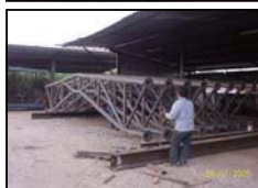
Fit-up roof truss
