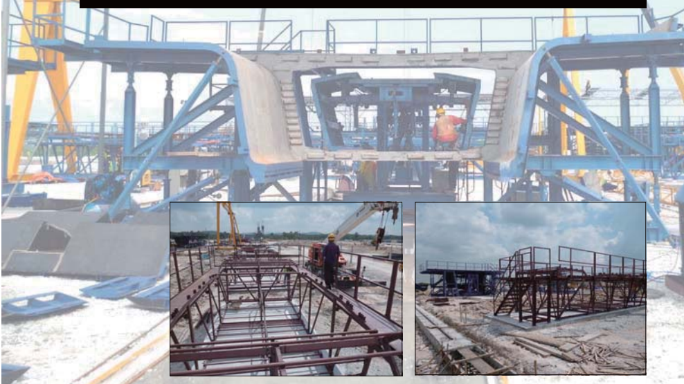
Rebar Jig on Site set up.
