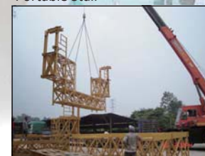
Loading At Our Storage Yard.
