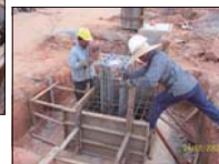
Holding Down Bolt Installation.
