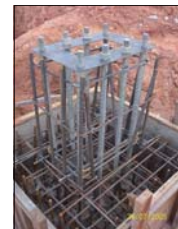
Holding Down Bolt Installation.
