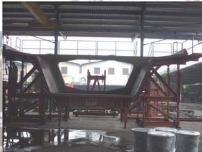
STEEL MOULD TRIAL ASSEMBLY
