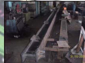
In house Fitting & welding works in progress.
