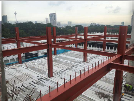
Steel Structure Column & Rafter Installation
