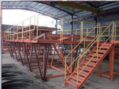
REBAR JIG TRIAL ASSEMBLY
