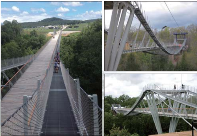
Site erection complete photos.
