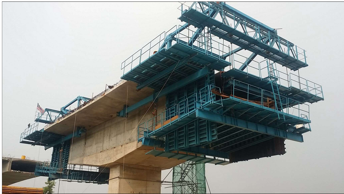
Form Traveller Erection At Site.
