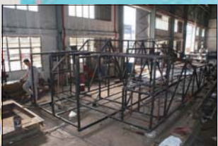
Steel Structure fabrication in progress.
