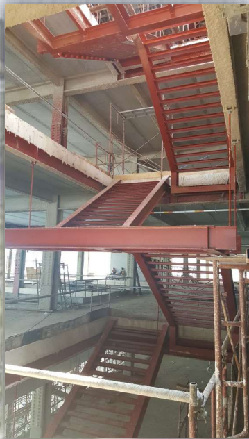
Suspension Staircase Installation
