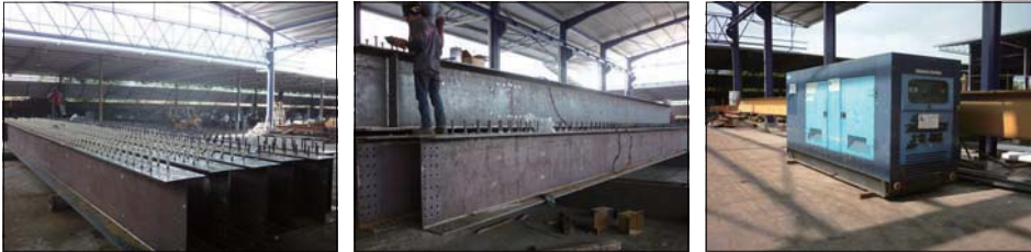
Stud welding on I Girder Beam.
