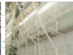
Trusses fitted to the wall by Chemical Anchor Bolts.
