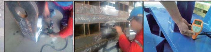
NDT test in progress
