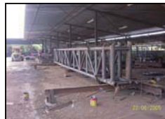
Fit-up roof truss
