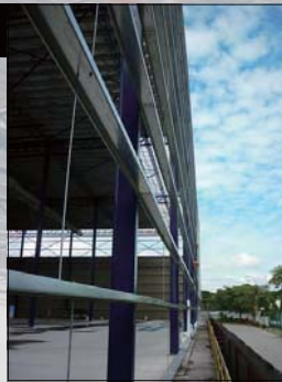
Site Erection works.
