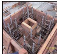
Holding Down Bolts Installation.
