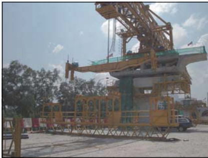
Stressing Gondola , At Site
