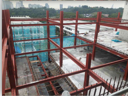
Steel Structure Column & Rafter Installation
