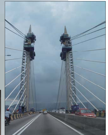
Working Platform Install on Bridge Pylon.
