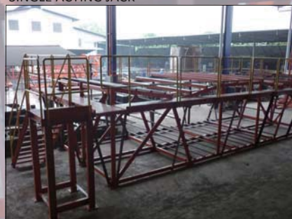
REBAR JIG TRIAL ASSEMBLY
