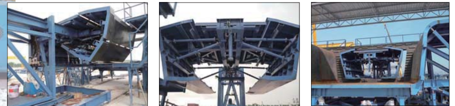
Inner form & hydraulic operation on Site set up.
