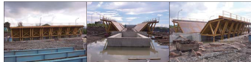
Steel Form Work.
